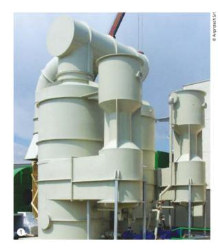
Figure 1: A Venturi scrubber-type wet filtration plant.
