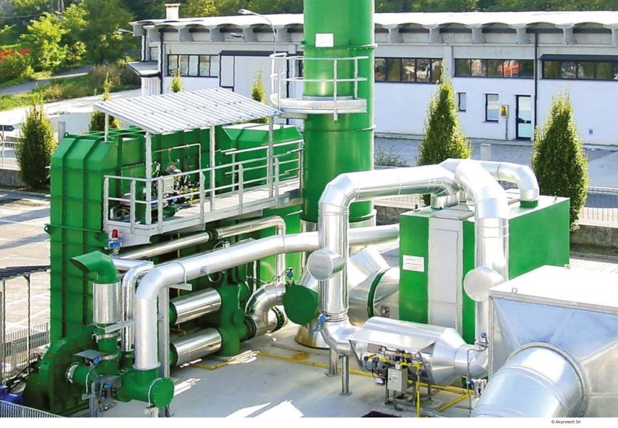
**Opening photo: Rotary concentrator + RTO system.**
